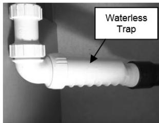
The waterless trap can be unscrewed from the water lines. A label has been placed near the location of the waste valve that reads as follows:
